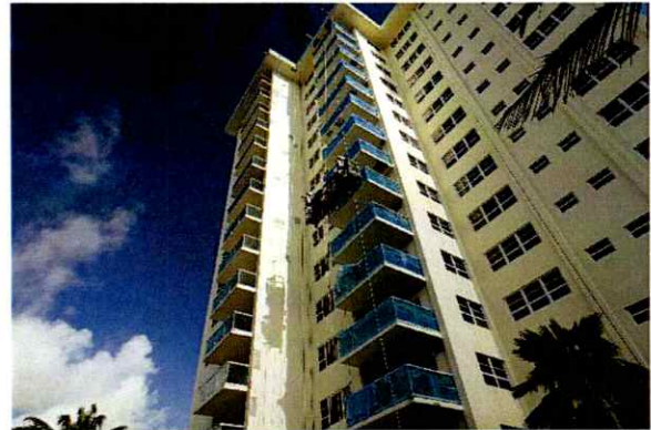
Figure 4: Repairs in Progress
