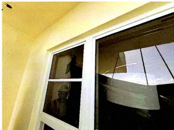
Figure 21: Sealant Was Observed in Good Condition.
