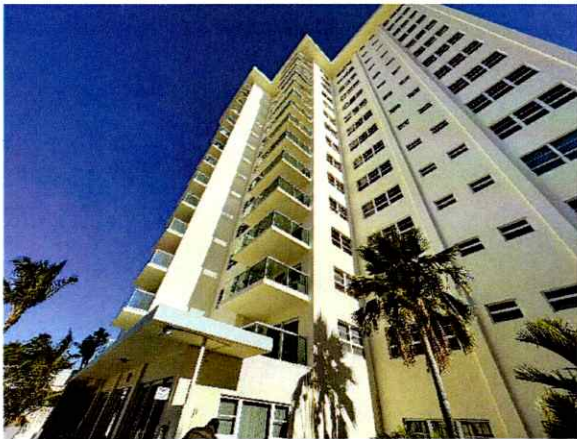
Figure 25: Condition of the Façade After Repairs
