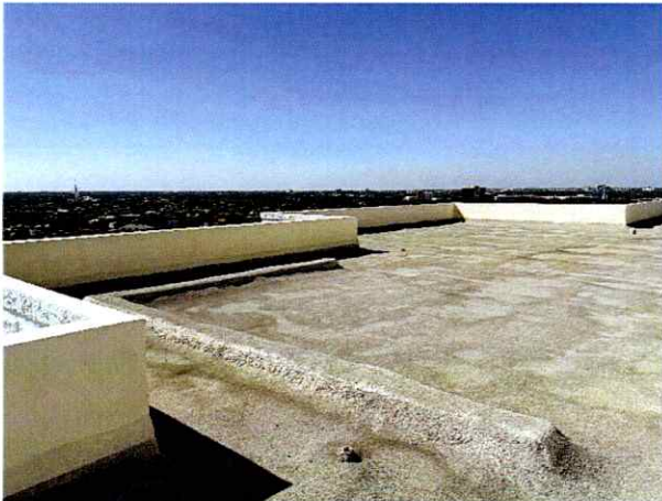
Figure 1: Roof Level Actual Condition
