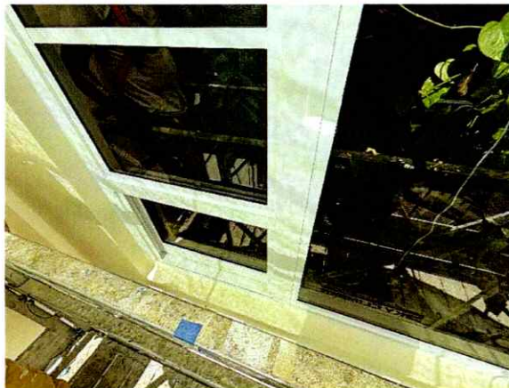
Figure 22: Sealant Was Observed in Good Condition.
