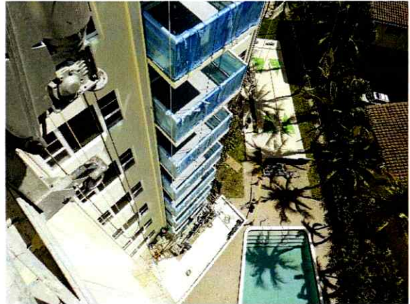
Figure 16: Waterproofing Application in Progress at Balconies.
