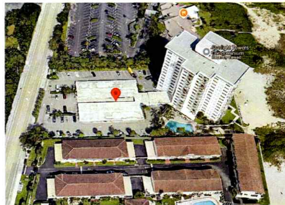
Figure 2: Aerial View of Building
