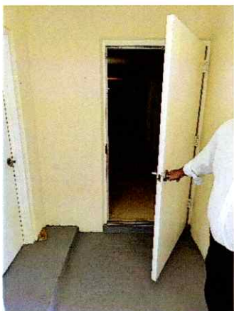
Figure 19: Metal Door for the Staircase.
