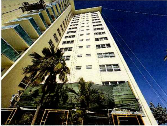
Figure 23: Condition of the Façade After Repairs
