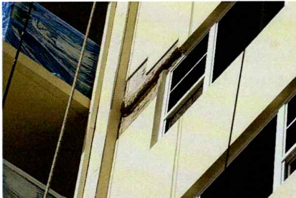
Figure 5: Repairs in Progress
