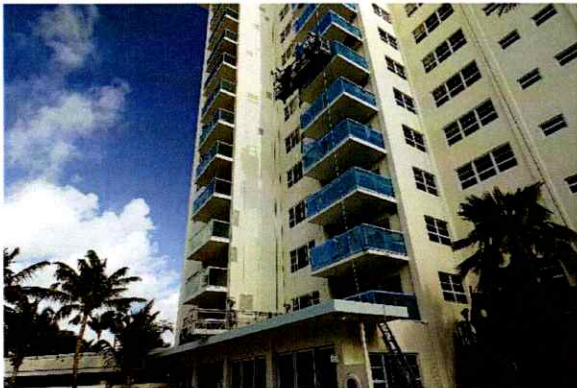
Figure 3: Repairs in Progress
