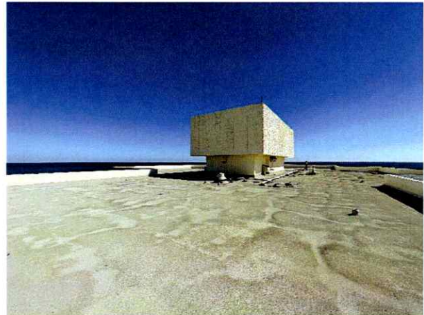
Figure 2: Roof Level Actual Condition.
