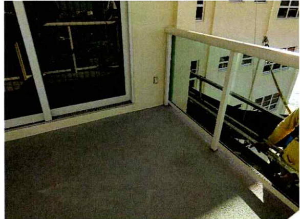
Figure 18: New Waterproofing Installed and Condition of Balcony Railing
