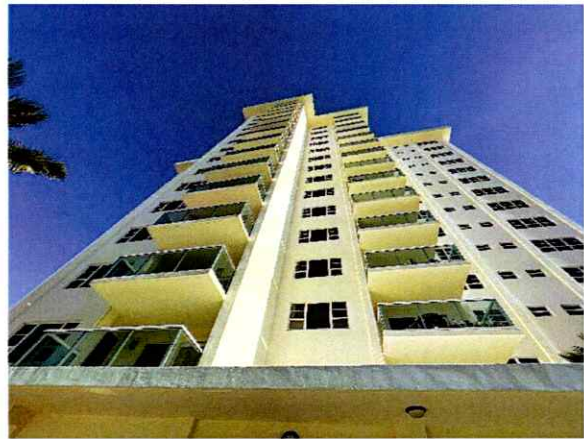
Figure 26: Condition of the Façade After Repairs
